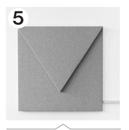
Measure the c/c distance from the edge of the panel that has already been installed. Then repeat stages 2–4.
