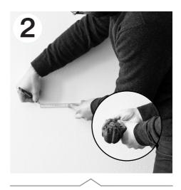
Measure c/c distances and mark the position of each anchor point.
