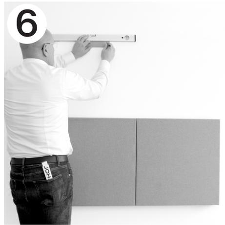
Repeat stages 3–5, using a carpenter's level to make sure that the panels are perfectly aligned.
