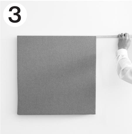
Measure c/c distances and screw the suspension rail into position. (Note that the rail has countersunk slots to facilitate vertical fine adjustment).
