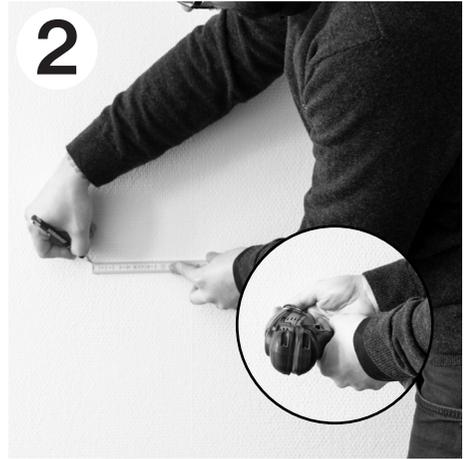
Measure the c/c distance for making the holes. Note that the c/c measurement differs according to the product chosen. This product is designed for magnetic suspension.
