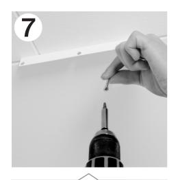
Mount the roof bracket with the supplied wooden screws. (Other attachment may be required for porous material).
