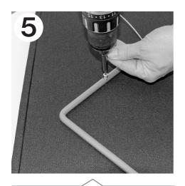
Use the two small wood screws supplied to secure the sound absorber in place on the bracket.
