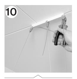
Surplus wire can be snipped off after the necessary adjustments have been made.
