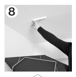
While supporting the sound absorber, hook it in place on the ceiling fitting, as shown in the photo
